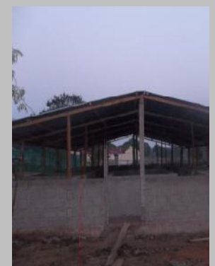
Photo Feature: the View of the Piggery under Construction
